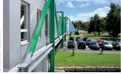
Zentrale Stetten a.k.M.
